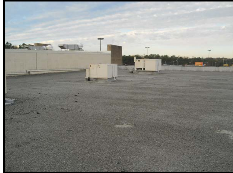
2 The roof of the former Cato Store (Store 1824).
