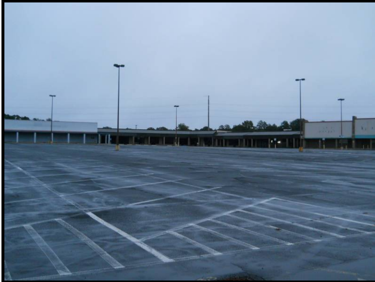
1 The subject building as seen looking roughly north from Wilson Road. The assessment did not include the former Winn-Dixie or Wal-Mart stores located at either end of the shopping center.
