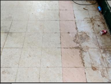
The 12" white and pink vinyl floor tile and associated mastic located in the garage tested negative for asbestos.
