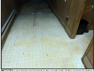
The tan linoleum located in the south side of the garage building tested negative for asbestos.
