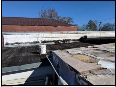
The asphalt rolled roofing tested negative for asbestos.
