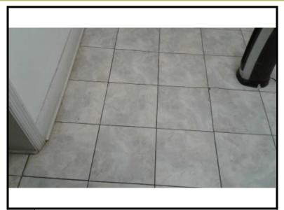
The tan/black mastic located beneath the self-adhesive vinyl floor tile in the women's restroom tested positive for asbestos (4% chrysotile).
