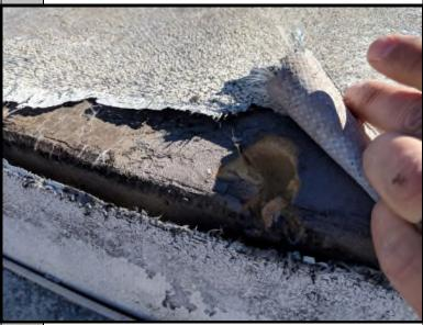
The cloth rolled roofing tested negative for asbestos.
