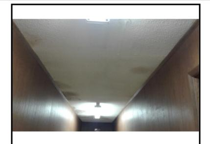
The spray-applied ceiling texture tested negative for asbestos.
